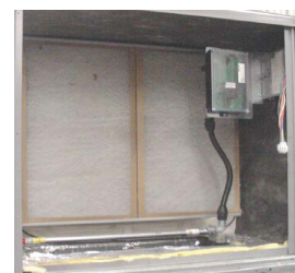
Fig. 25 - Return Air Sensor Operating Position
