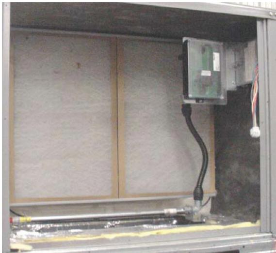
**Fig. 23 — Return Air Sensor Operating Position**
