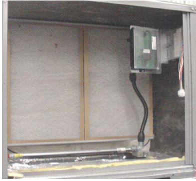
Fig. 41 - Return Air Sensor Operating Position
