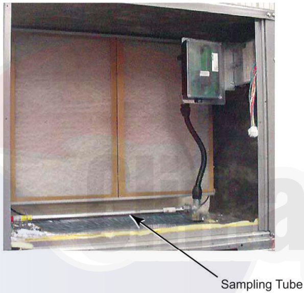
Fig. 96 — Return Air Smoke Detector, Shipping Position
